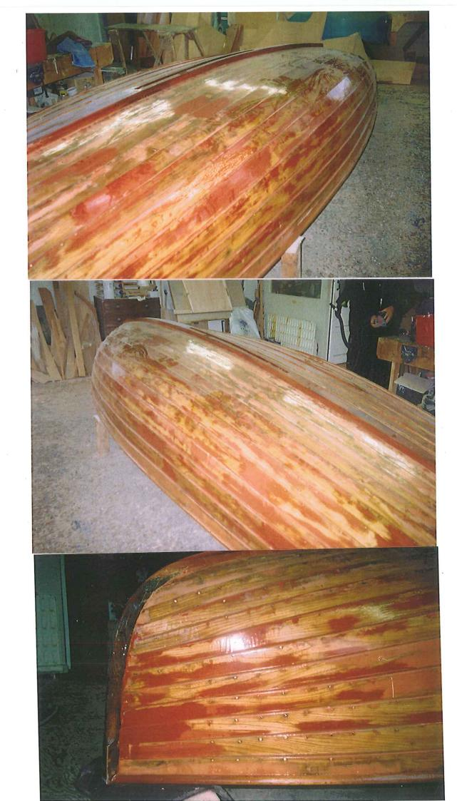
22. Paint the hull. For one colour all over with boot-top / waterline coachline, a good production method is as follows:-
